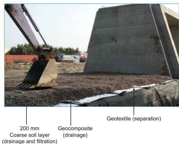
Figure 2. GRS wall construction: provision of a 200 mm thick layer of coarse soil cushion above drainage layers prior to placing of locally available backfill soil (courtesy of Gold-Joint Industry Company)
